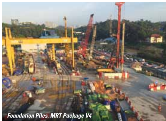
Foundation Piles, LRT Extensions at E6 Central Link
